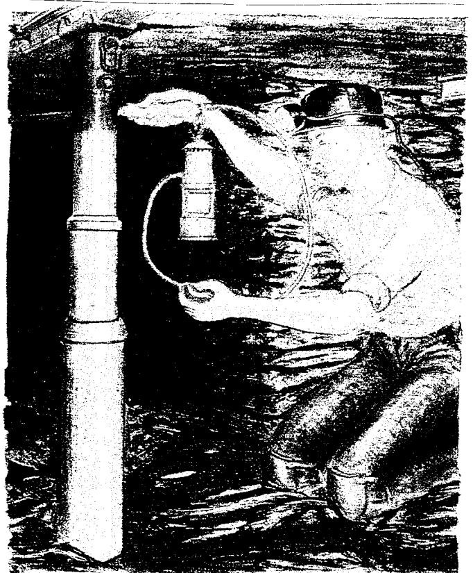
Testing for gas in the waste with a Probe Lamp.
